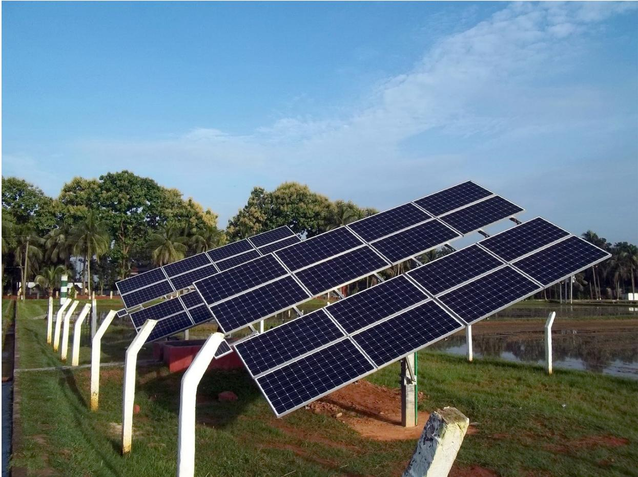
If the Sun can be tracked according to these math models, the maximum possible harvest can be obtained. However, some form of solar-tracking structures will be needed. An example of sun tracking system is shown above. This was designed by a friend of mine and myself back in 2012. He designed the mechanical section while I added the intelligence in form of embedded-system coding and tracking controller design.
